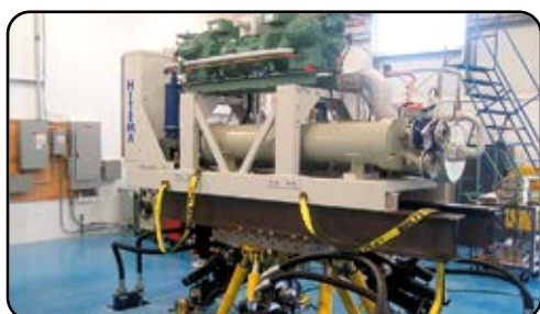
* Seismic test, installed in Canada, 300 kW
