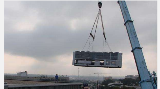
COUNTRY OF INSTALLATION: Wisconsin, United States MODEL: EEf.1100 with freecooling and inverter screw compressors NOMINAL COOLING CAPACITY: 1132 kW
