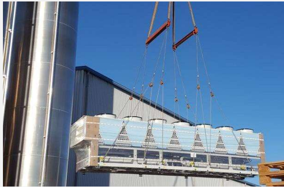
COUNTRY OF INSTALLATION: Spain MODEL: ISV.910 NOMINAL COOLING CAPACITY: 850 kW
