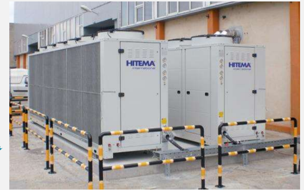
COUNTRY OF INSTALLATION: Moscow, Russia MODEL: No. 2 pcs ENRF.370 with freecooling NOMINAL COOLING CAPACITY: 2X365 kW
