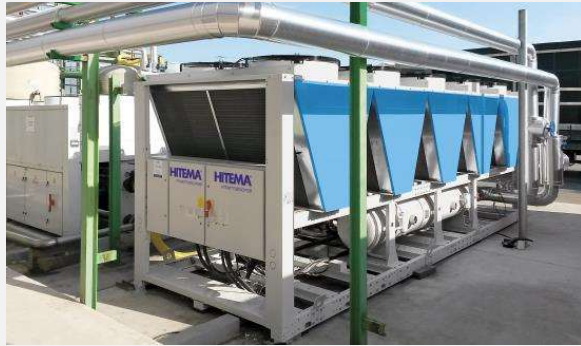
COUNTRY OF INSTALLATION: Ukraine MODEL: SBS.720 NOMINAL COOLING CAPACITY: 718 kW
