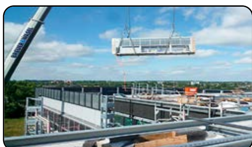
* Chiller installed in Dusseldorf, Germany, 820 kW
