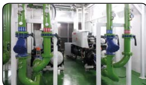
* Chiller installed in Dusseldorf, Germany, 820 kW
